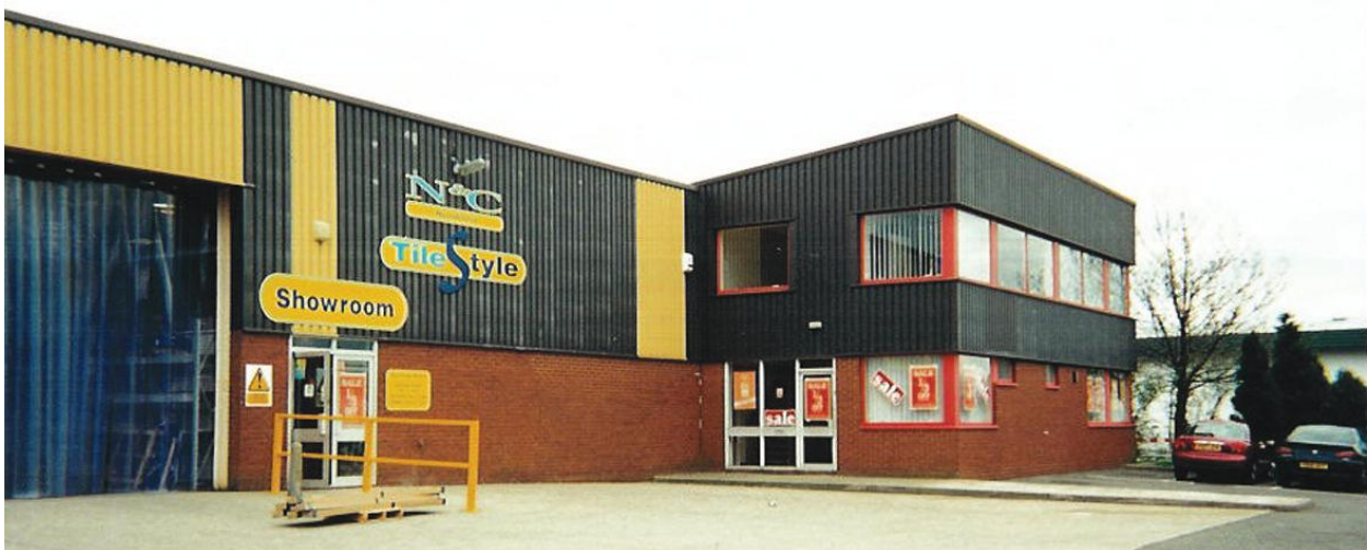
Distribution and retail unit, Southampton
